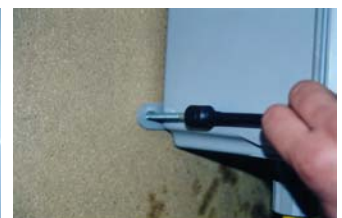
Anchor Controller to Wall
