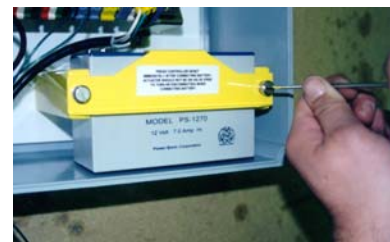
Securing battery
